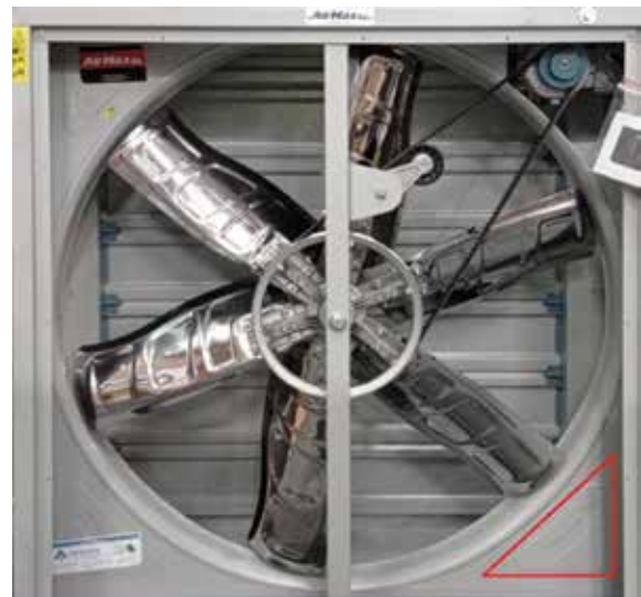
Figure 8. Arrows indicating the correct direction of rotation of the propeller. Check that the shutters open when the fan starts to turn. If this does not happen and the check from the previous list has already been carried out where it is checked that the shutter mechanism is moving freely, then the fan is turning in the opposite direction to that required.
